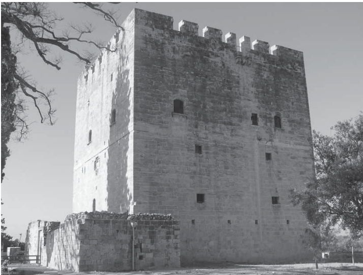
Fig. 80: Kolossi, keep, general view of the exterior, looking southwest [M. Olympios].
